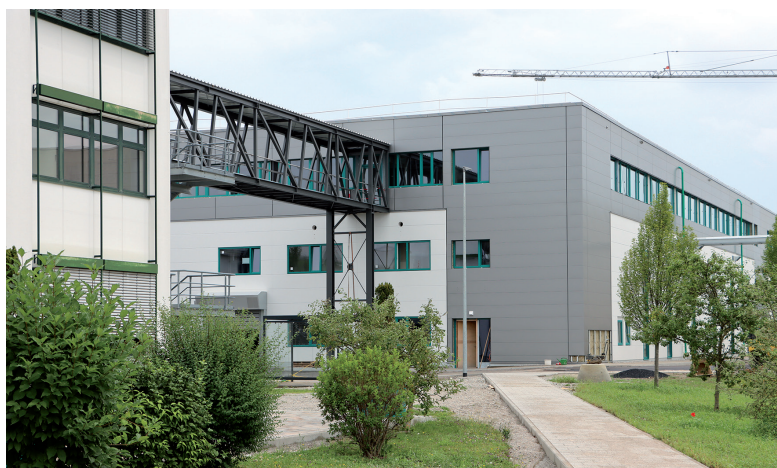
Fig. 1: The various buildings are connected by a glazed bridge. The special glazing of the windows helps to contain the transmission heat loss.
