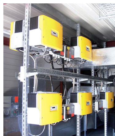
Fig. 3: Photovoltaic-inverter for grid supply
