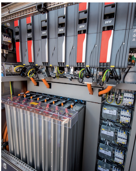
Fig. 5: The control cabinet contains two power supply modules and four single-axis modules. The black storage unit and its double-layer capacitor modules is installed underneath.
