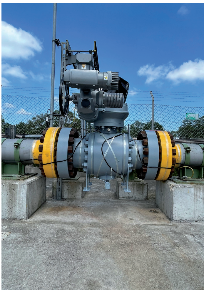
Fig. 1: Control ball valve 12" cl1500 as main feed-in and withdrawal control valve for natural gas cavern storage in Etzel (with trace heating without insulation in the installation phase)
