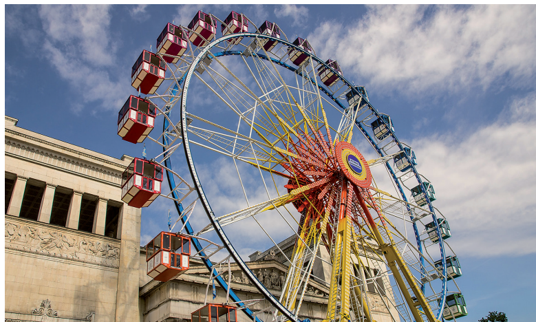
Fig. 2: Gerstlauer Amusement Rides manufactures its Giant Wheels in both stationary and transportable versions (shown here). They also come in different sizes. One particularly striking feature of Giant Wheel RR 40 is that it is designed with four columns instead of the usual eight. This provides greater transparency and an elegant look.
